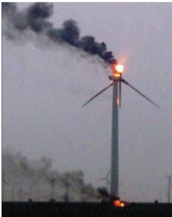
Photo 1: consequences of lightning strikes on wind turbines
