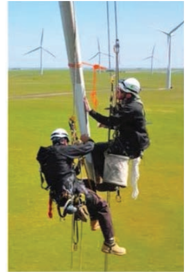
Photo 5: Blade damage repair
