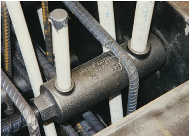
Interlok Grout-Filled Precast Splicing System
