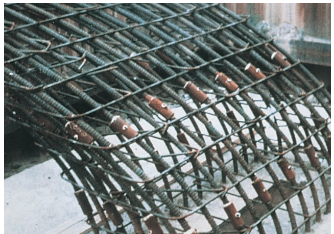
Cadweld Metal-Filled Splicing System
