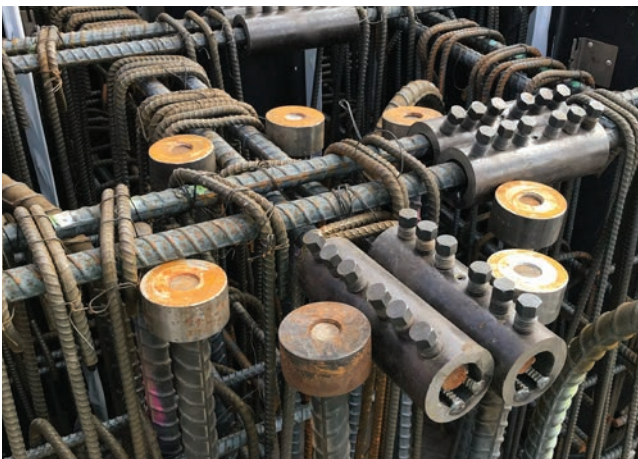
Connect Shear Bolt Splicing System
