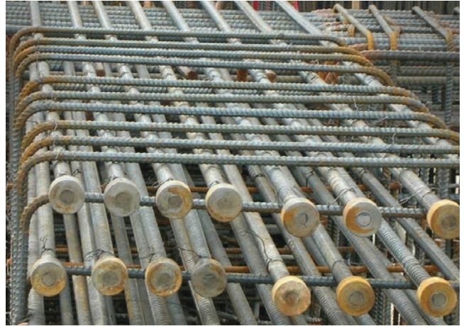
Taper-Threaded Terminators and Mechanical Anchors
